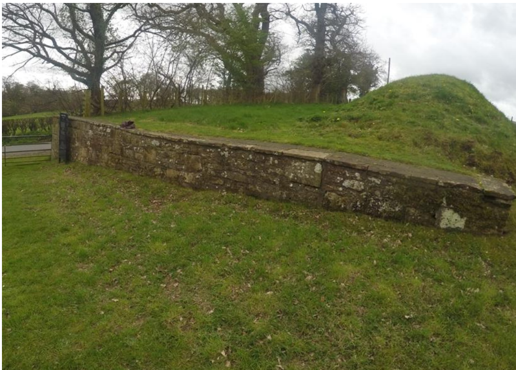
Photo 80: Abutment, near Dovecote Bridge, with 20 metres of (earth covered) wall on top. Turret 55B is located nearby although there's nothing visible on the surface.
