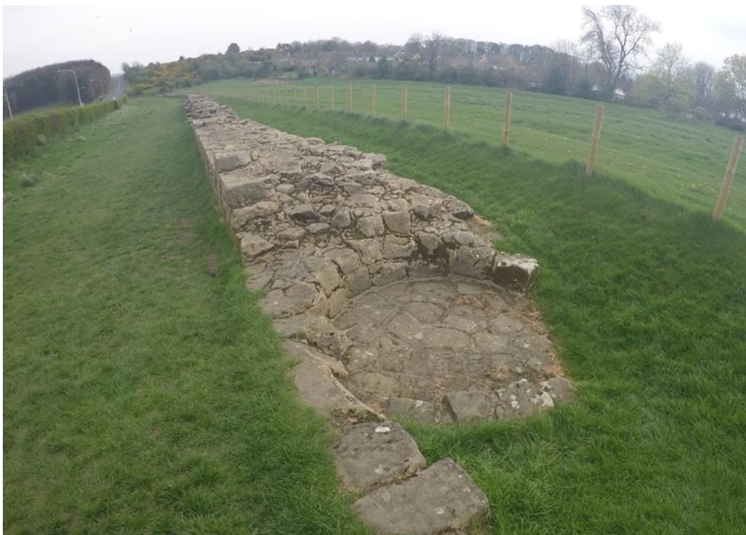
Photo 10: First major piece of wall @ Heddon-on-the-Wall. Circular feature in the wall is an Oven/Kiln which was built into the wall at a much later date than its original construction. An Example of Broad Wall on Broad Foundations.
