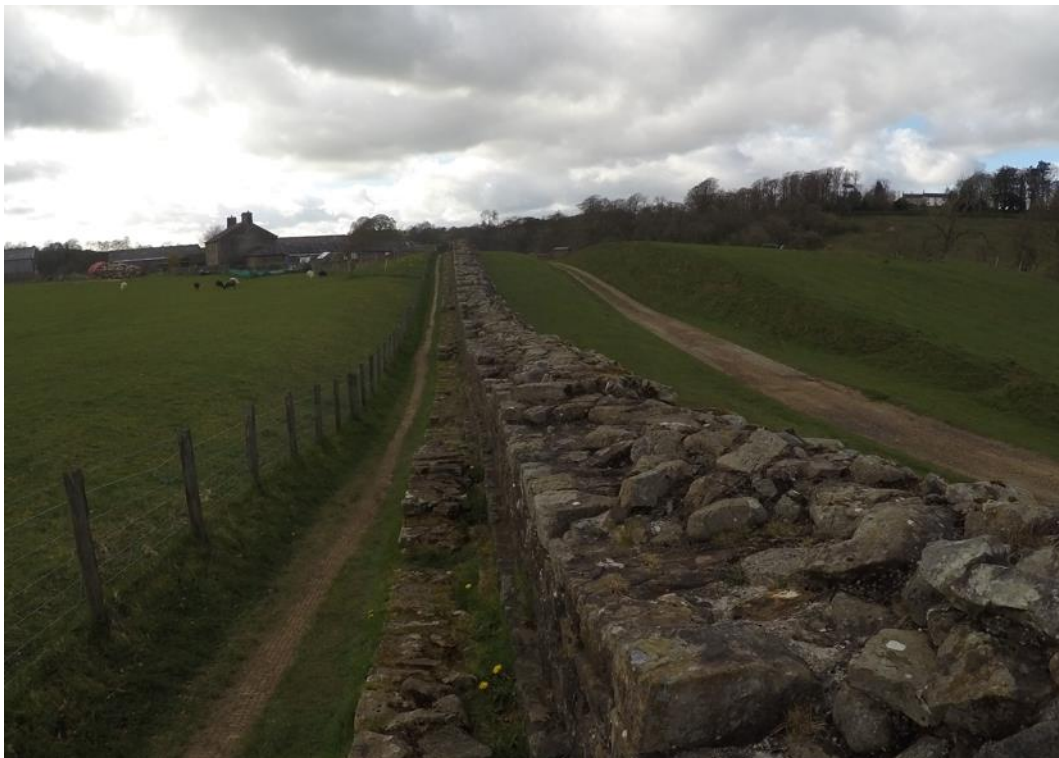
Photo 68: Example of narrow wall on broad foundations. Broad foundations stop at Willowford, with only narrow wall on narrow foundations after this point.
